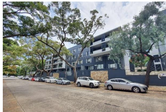
Figure 9 Hunter Street facing West
